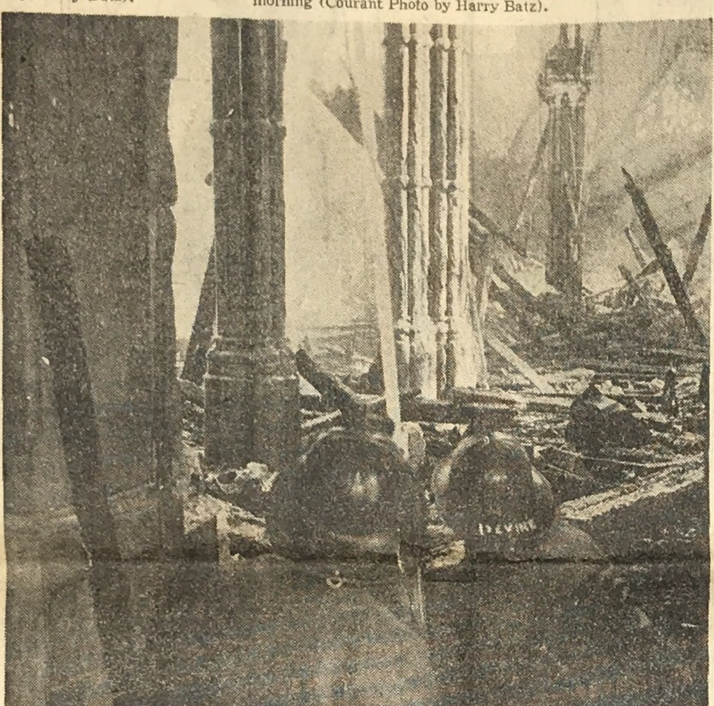
STILL DRENCH RUINS: Hoses, lines continued to pour water into the smoldering Cathedral Tuesday. These two firemen are in a side entrance looking across the front of the church where rubble is piled around the scarred pillars (Courant Photo by Harry Batz).
